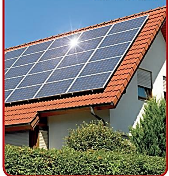
Photovoltaic (solar) panels
