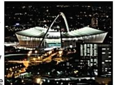
Energy to light offices and sport stadiums
